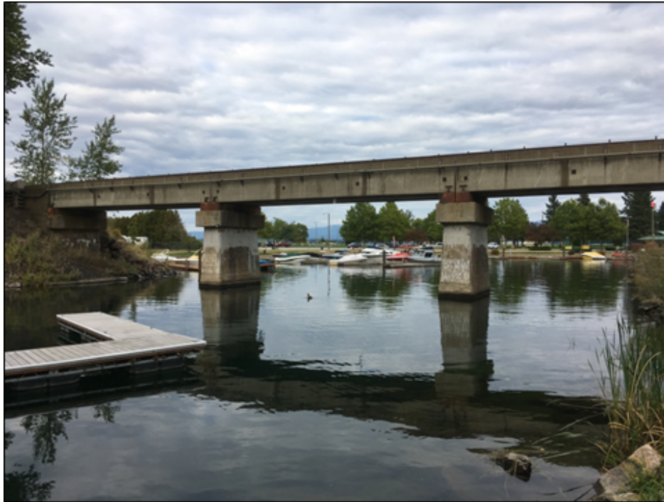
Bridge 3.1, West Elevation
