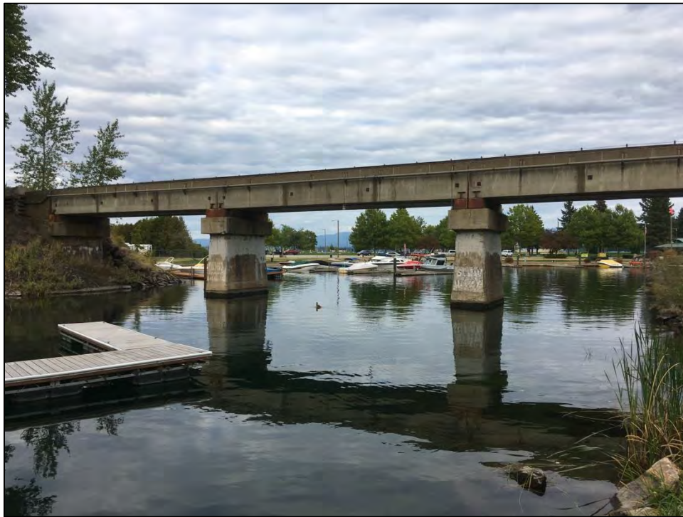
Figure 32. BNSF Bridge 3.1, West Elevation
