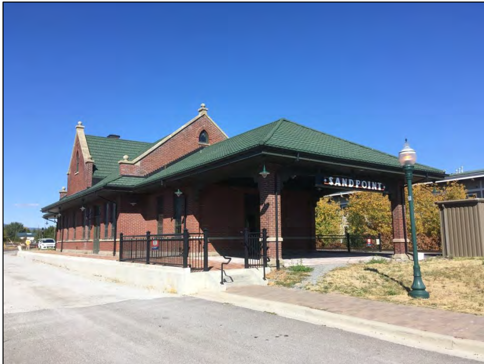
Figure 26. Northern Pacific Depot, South and West Elevations
