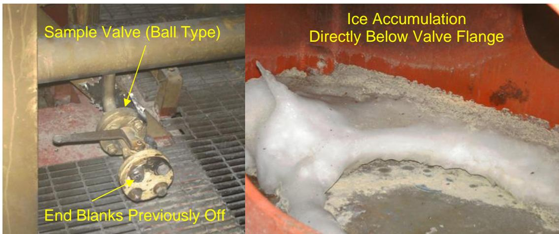
been removed and left off. Investigators were told that the Cargo Engineer regularly made rounds to manually drain the hydrates to the bucket in order to prevent the freezing of the expansion valve. However, no buckets were found and significant accumulations of ice were noted in the bilge areas below the same sample point for two of the three liquid line drains.
