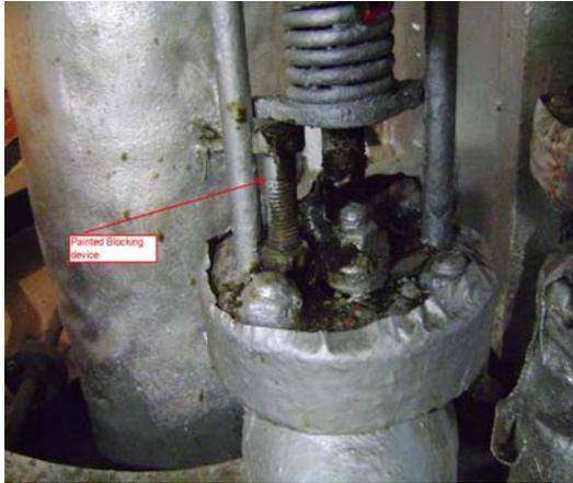
QCV blocked utilizing a bolt to hold in the open position. (Note: the painted portion on the bolt indicating possible long term condition.)
