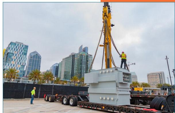
Shore Power Installation at Port of San Diego
