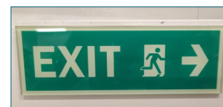
Photoluminescent exit sign
