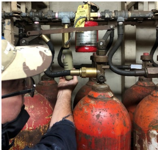
Pilot Bottle Actuation Lever Under Load and Activated
