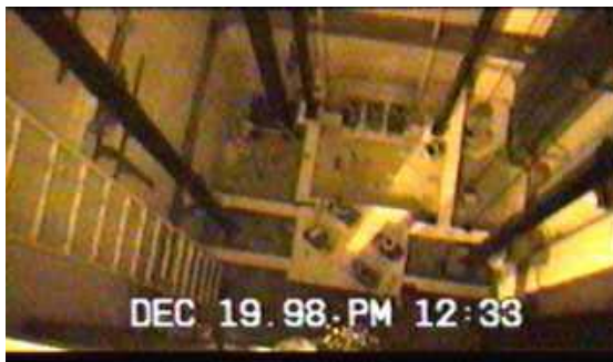
Top down view of a flooded elevator shaft and top of elevator.
