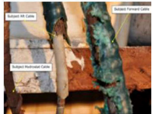
Figure 49: Lifeboat No. 6's aft hook control cable after the casualty. The aft cable is in the center of the picture. Credit: CG.
