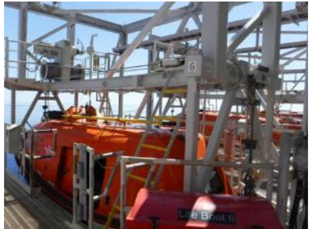
Figure 7: Lifeboat Station No. 6 davit. Figure depicts raised landing where winch is located. Credit: Palfinger, dated May 2015.
