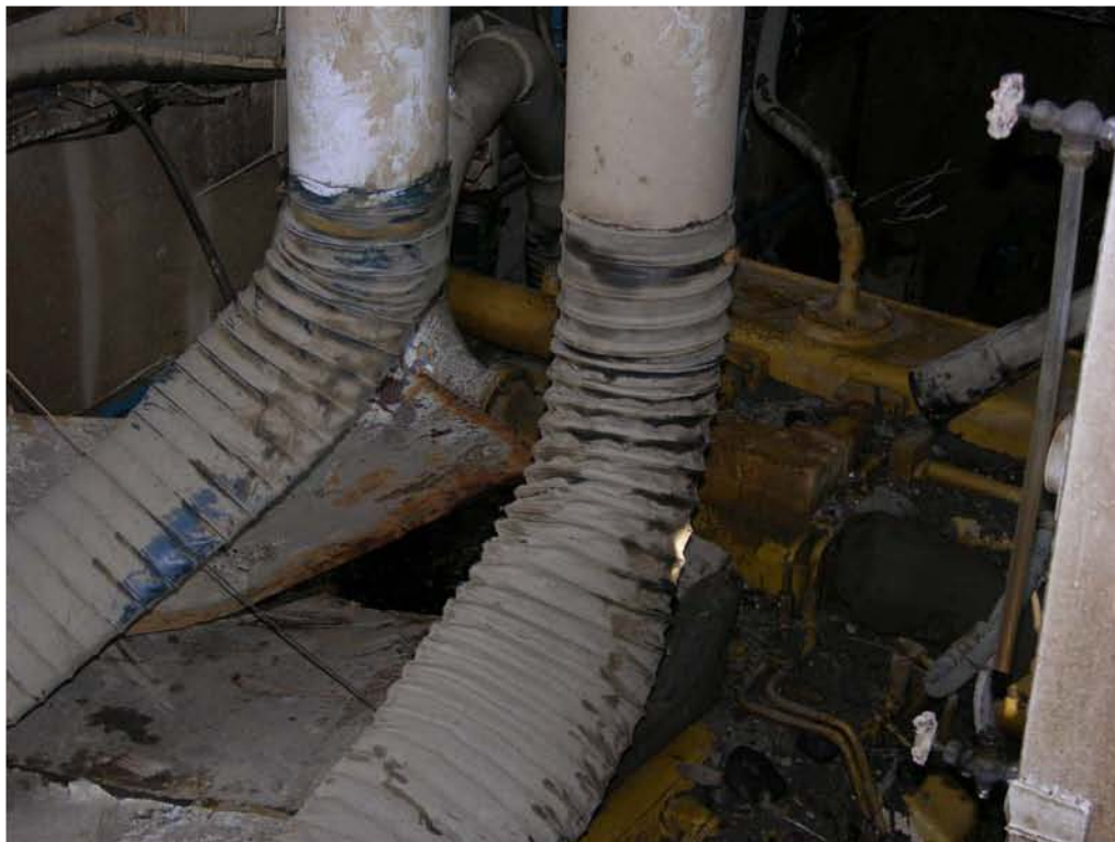
Collapsed PVC hoses at the steel piping connection from air filter housing.
