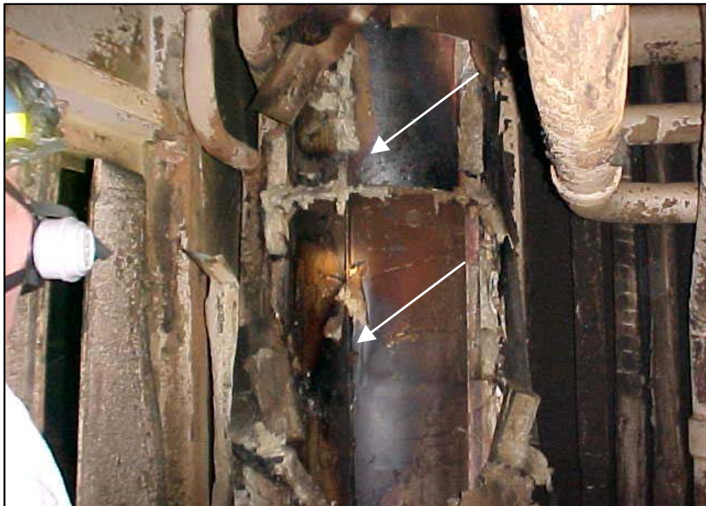
Picture 7: Auxiliary Boiler Exhaust Stack (between Main Deck and 01 Level) [Arrows depict location of black stains]
