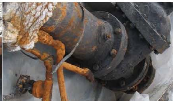
Figure 5-30: Starboard header with heat trace piping Figure 5-31: Port header with heat trace piping
