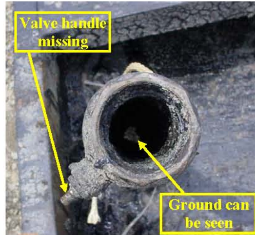
Figure 5-16: Standpipe penetrates remnant of deck plating
