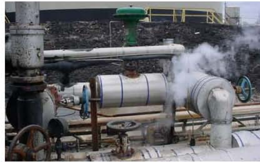
Figure 8-6: Steam supply control valve for tanks 515/516
