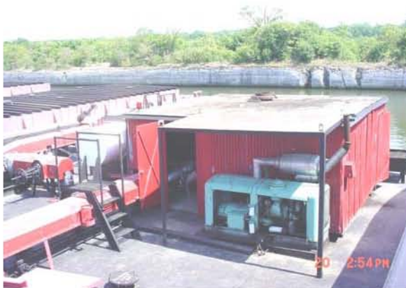
Figure 5-36: EMC 472 Vapor thermal fluid heater
