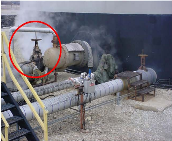
Figure 9-3: Main suction valve on storage tank 516
