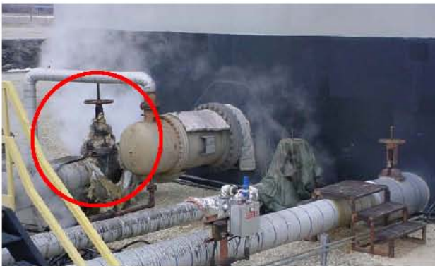
Figure 8-7: Main suction valve on storage tank 516
