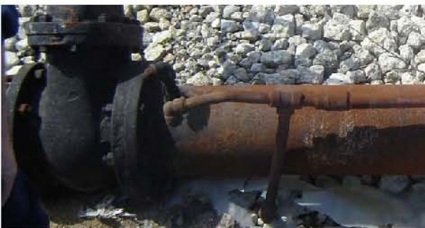
Figure 5-30: Starboard header with heat trace piping Figure 5-31: Port header with heat trace piping
