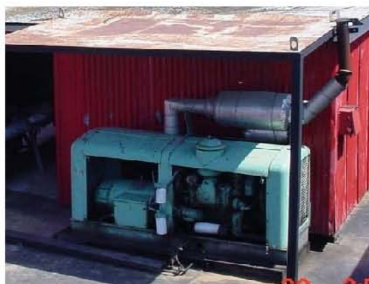
Figure 5-34: EMC 472 generator/4V-71 Detroit Diesel
