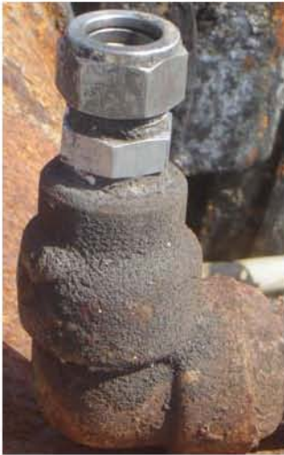
Figure 5-28: Header compression fitting
