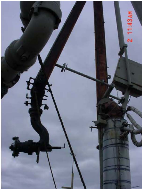
Figure 9-2: CSO Loading arm at ExxonMobil Pg.1221).
