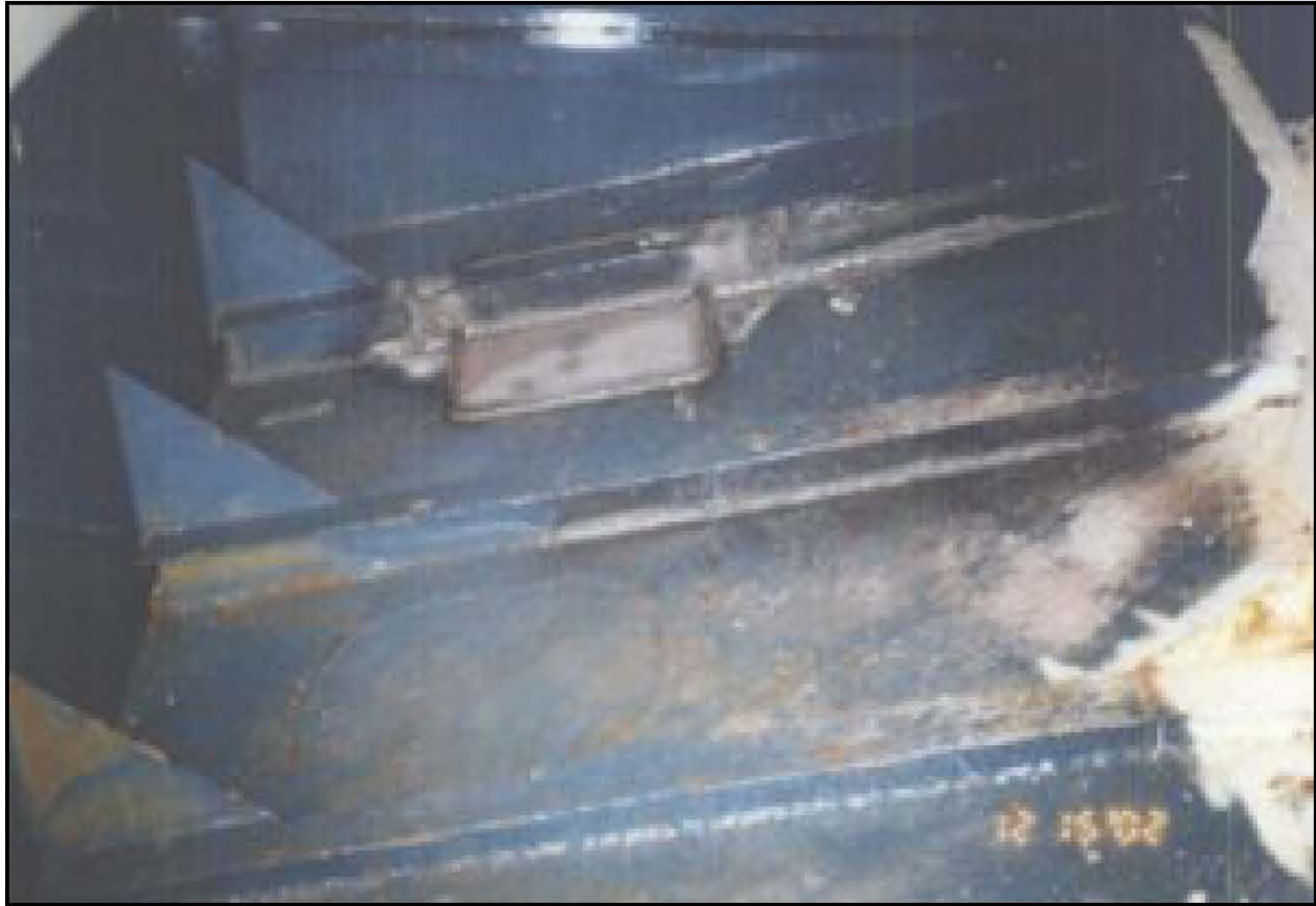
Figure 21: Photograph taken inside of potable water tank showing doubler.
