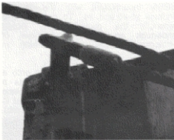
Twisted eye/hook connection
