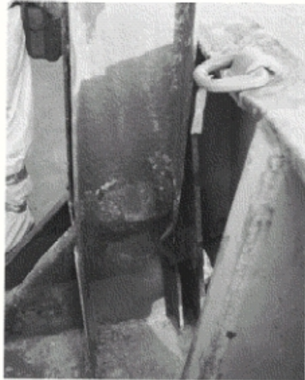
Compression damage at bottom of pedestal
