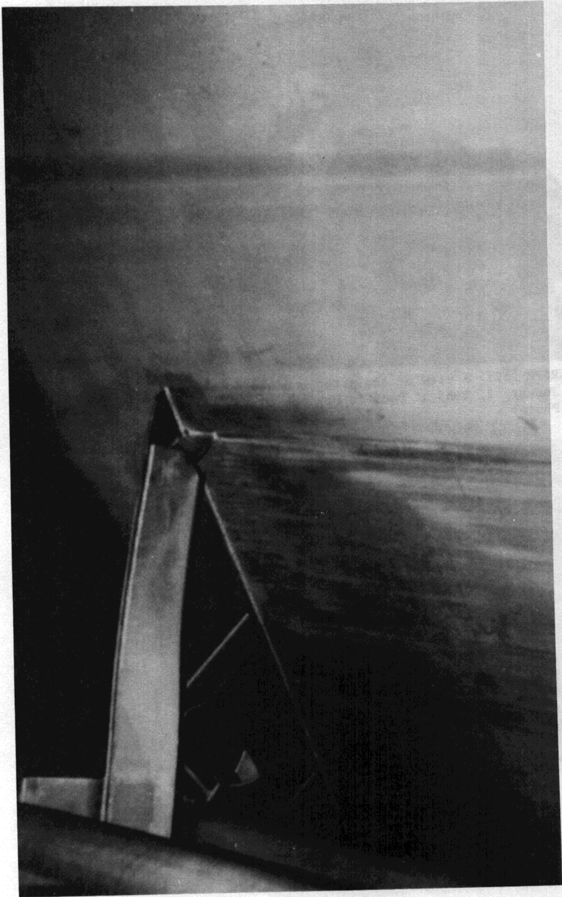
PHOTOGRAPH #11: A detailed view showing the hole from the 5CP side. It is located below a horizontal stiffener plate and behind a cutout in a vertical gusset plate which are part of a horizontal corner bracket. (FaAA Photo taken November 19, 1985)
