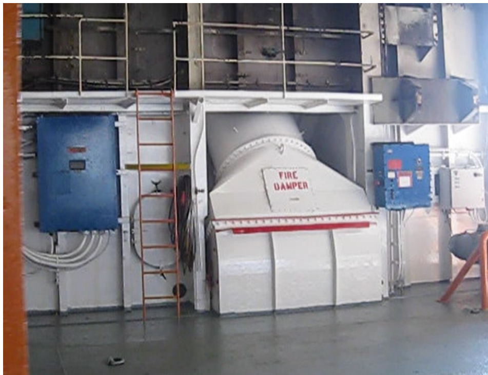
Figure 6-12: Hold 3 ventilation supply fan and fire damper enclosure, frames 141-144 starboard, 2 nd deck. Screen capture from video taken September 2008 provided by Tote, Inc.
