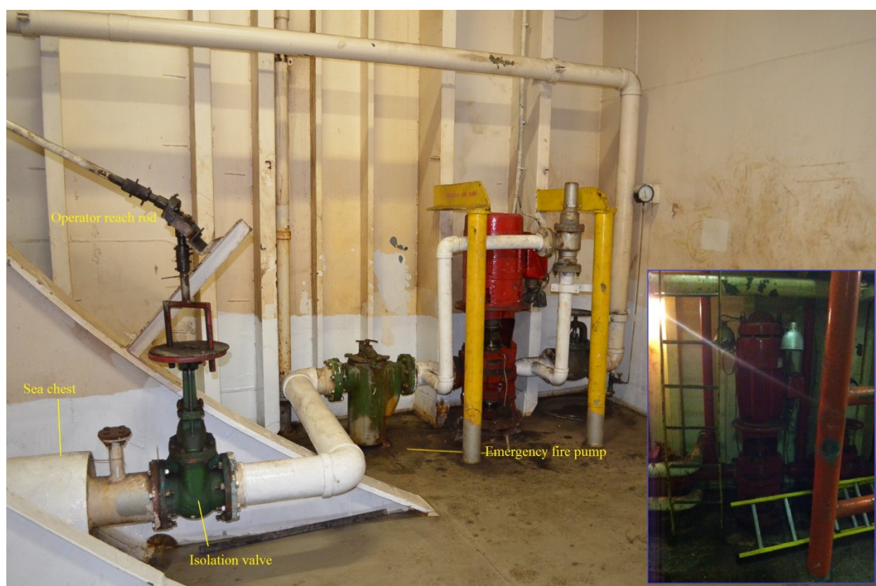
Figure 6-7: Emergency fire pump station in Hold 3, aft starboard 4 th deck (tanktop, innerbottom), showing the sea chest, isolation valve, and manual remote operator on sister vessel EL YUNQUE (EL FARO similar but not identical). Inset photo shows part of the arrangement onboard EL FARO. USCG photo with Tote, Inc. photo inset.
