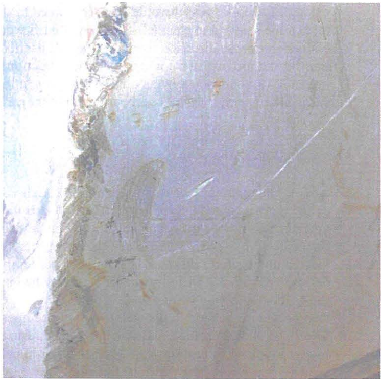
Figure 10. Photograph of SEA MULE damaged bow taken December 1, 2022 by USCG
