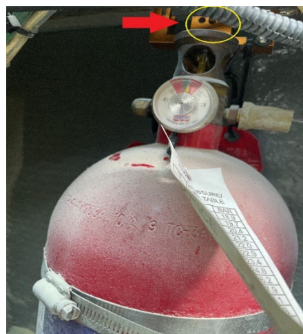
Figure 4 Sea-Fire NFD 500 Series safety pin placement
