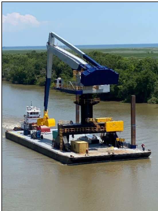
Fig 1: Barge with crane loaded on board.
