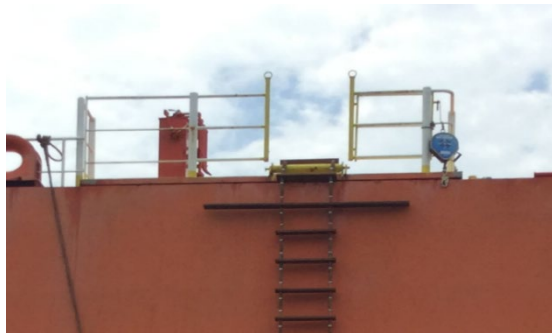
Figure 2: Gap in handholds appear to accommodate spreader.
