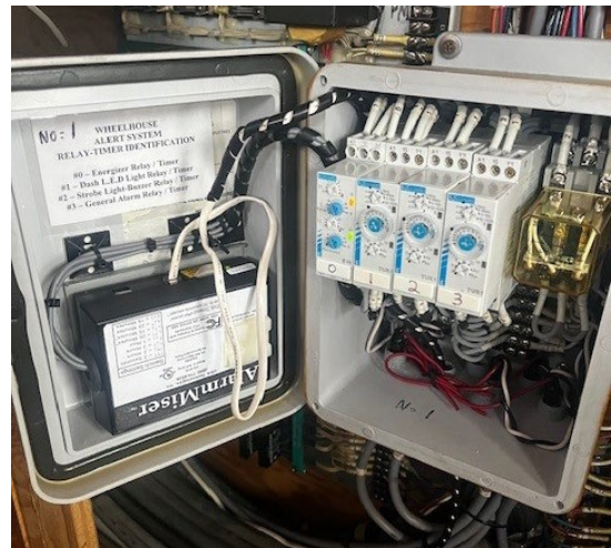
Figure 3: Pilothouse Alerter System Timer Adjustment Panel.
