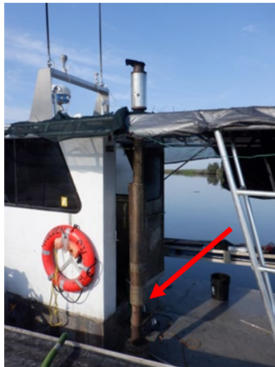
Main Engine Dry Exhaust
