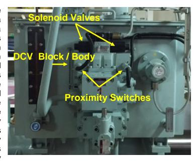
and required replacement. Ignoring the problem meant that although the rudder moved as expected in these two cases, the lack of properly functioning proximity switches might result in a failure to detect if the rudder had not moved, since crewmembers had trained themselves to ignore the alarm.
