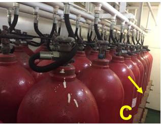
As a result of the inspection the vessel was detained until these and other identified deficiencies identified were corrected. During a reinspection of the vessel to clear the deficiencies, it was discovered that the servicing organization that replaced the hoses, installed several new hoses in a similar orientation that maintained excessive stress on the hoses. That issue was subsequently rectified by rotating the bottles.
