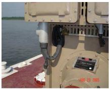
An acceptable engine control unit (ECU) enclosure is shown here with a sealing compound installed in a proper cable gland. Sealing compound poured in the conduit or cable seal fitting should surround each individual insulated conductor and the outer jacket of the cable, unless the cable is gas tight. Cables should be prevented from being pulled out of the conduit or cable seal fitting.
