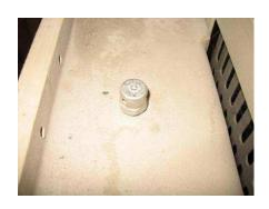
Batteries should be placed in explosion proof enclosures and should have an approved breather installed on top.
