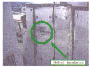
with similar insulation installations should remove this material as soon as possible. The Coast Guard's primary concern with the use of polystyrene insulation is that a minor fire, which normally could be easily contained, may suddenly result in rapid flame spread and large amounts of black smoke which could disable or trap crew members. Additionally, heat generated by the combustion of polystyrene insulation could ignite other materials, resulting in the loss of a vessel.
