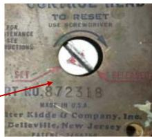
The slot and arrow indicator on the released component above aligns with the status of the CO<sub>2</sub> bottle.
