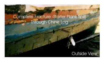
As the hull continues to work, these checks can widen into fractures, with the worst case of both the chine log and the outside starter plank fracturing all the all the way through.
