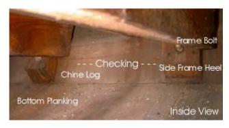
Initial indications include shallow checking of the face of the chine log on the inside or on the face of the starter plank on the outside "bolt to bolt."
