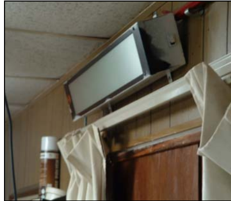
Figure 39. Green light installed over doorway to prevent circadian rhythm disruption.
