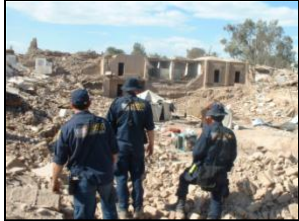
(12/23/03) Fairfax County US&R squad inspect earthquake damage in Bam, Iran. (Photo by Marty Bahamonde/FEMA)
