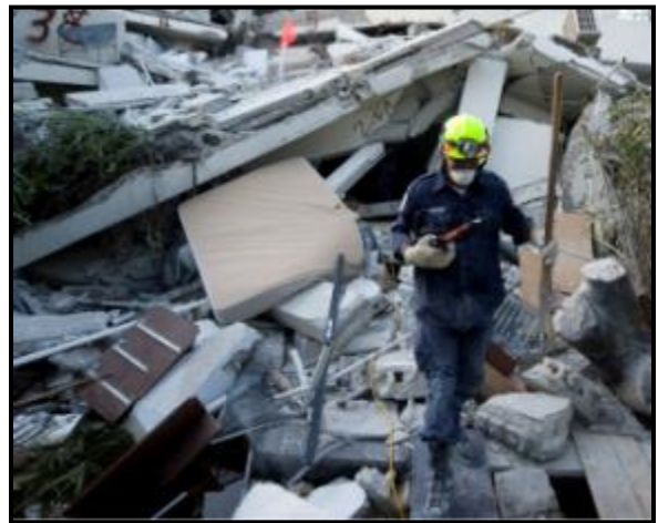
(01/14/10) Members of Fairfax County US&R Task Force conduct a rescue operation in a collapsed section of the Hotel Montana, Port-au-Prince, Haiti, during a search for survivors of a 7.0 magnitude earthquake. Eight people were rescued from the hotel rubble. (Photo: Chief Petty Officer Joshua Kelsey/USCG)
