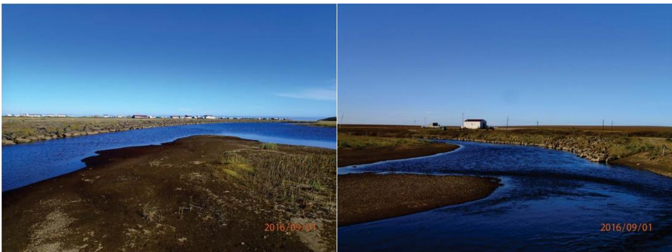
Figures 3 and 4. Revetments Along Airport Road
