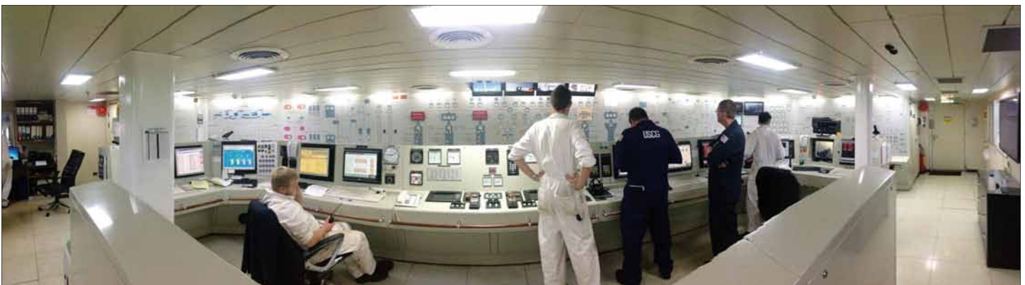
Inspections, such as this one of an engine control room, are imperative to discovering deficiencies. U.S. Coast Guard photo by ENS Jordan Ortiz.
