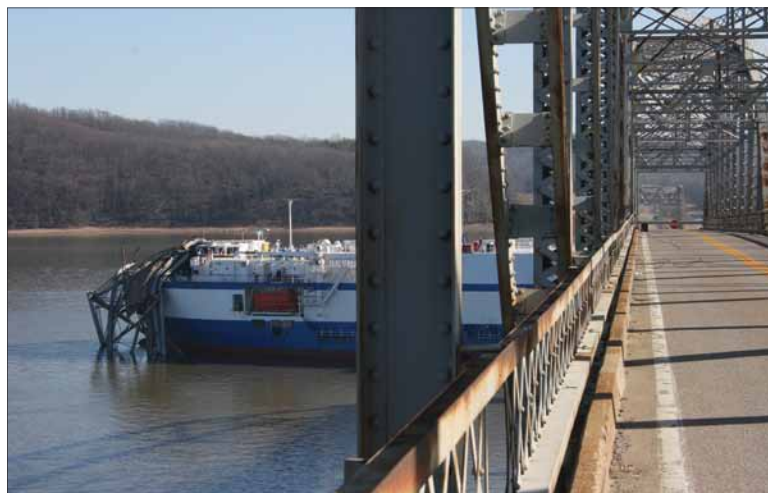
The M/V Delta Mariner anchored to the river bottom in Kentucky Lake on the Tennessee River with the span of the Eggner’s Ferry Bridge draped across her bow. Photo courtesy of the National Transportation Safety Board.
