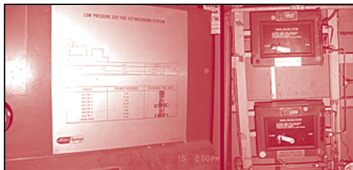
Valve release diagram and valve releases for engine room and hold 3.
