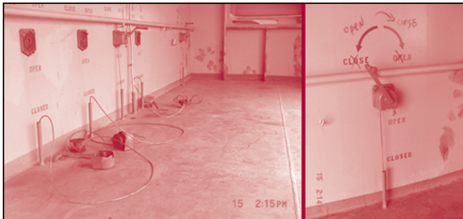
Broken damper controls and improperly marked control.
