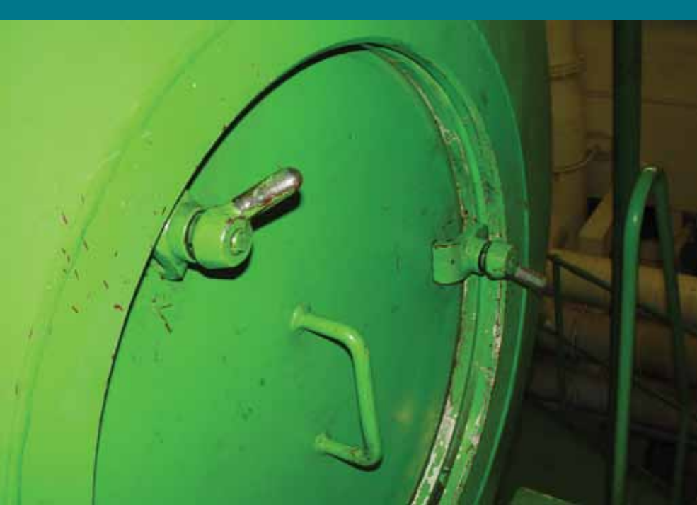
Forward end of the scavenge air receiver.
