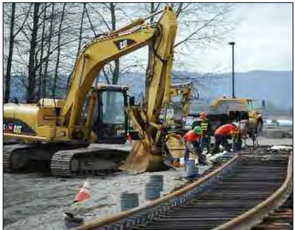
Workers prepare to install a rail switch at the Port of Vancouver. Photo courtesy of Ms. Katie Odem, Port of Vancouver.
