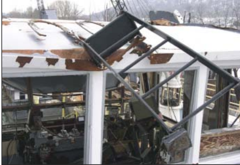
Post-casualty photograph of the ladder leading to the top of the pilothouse used by the deckhand to secure himself and the captain until they were rescued.
