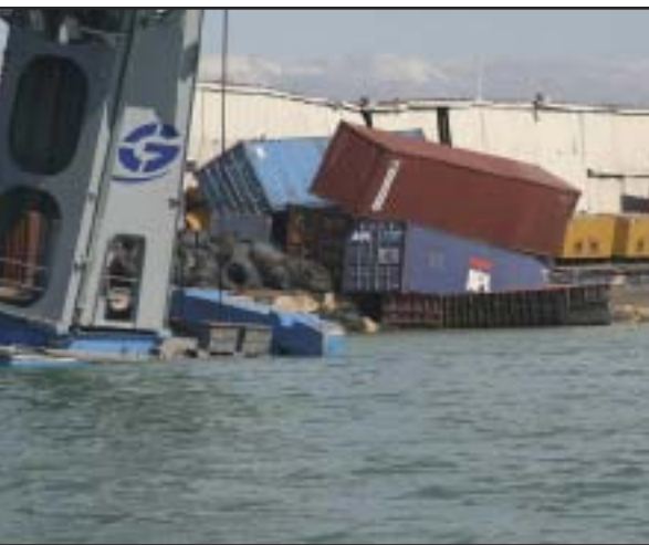
Damage to the port hampered delivery of relief supplies. U.S. Coast Guard and other responders worked to survey and repair the port infrastructure. U.S. Coast Guard photo.
