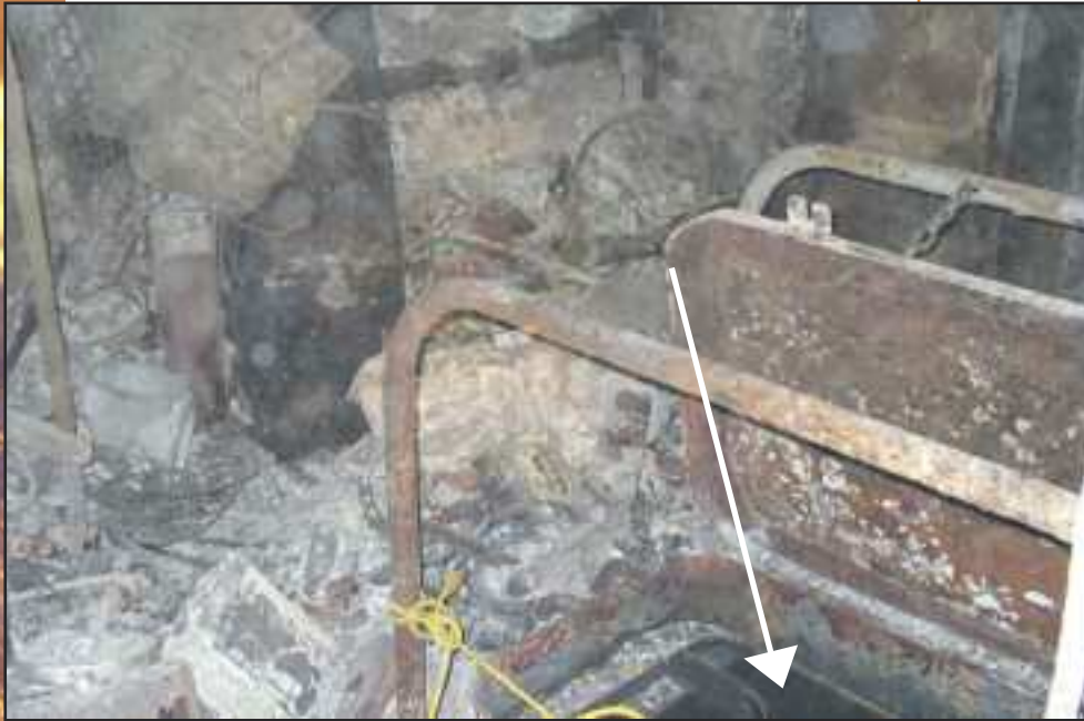
The storage area where the chief engineer first noticed the fire. The bottom right of the picture shows the hatch leading to the bow thruster room.
