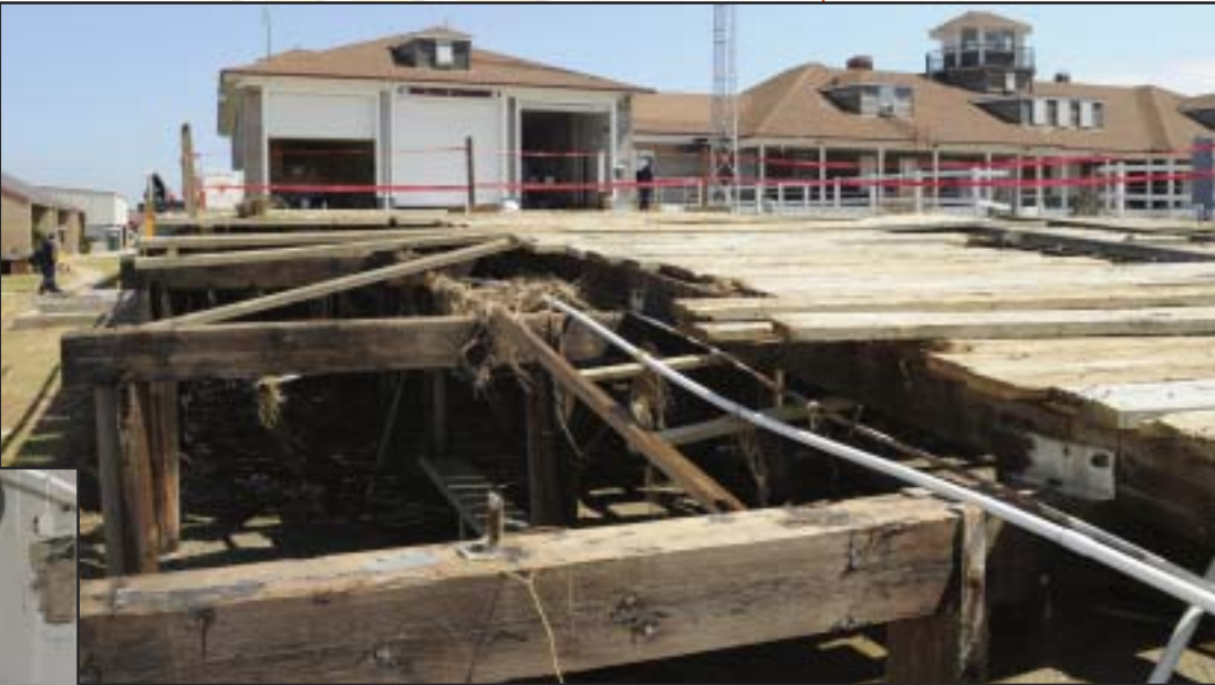
Station Galveston sustained major damage following Hurricane Ike. USCG photos by Petty Officer Kevin Rofidal.
