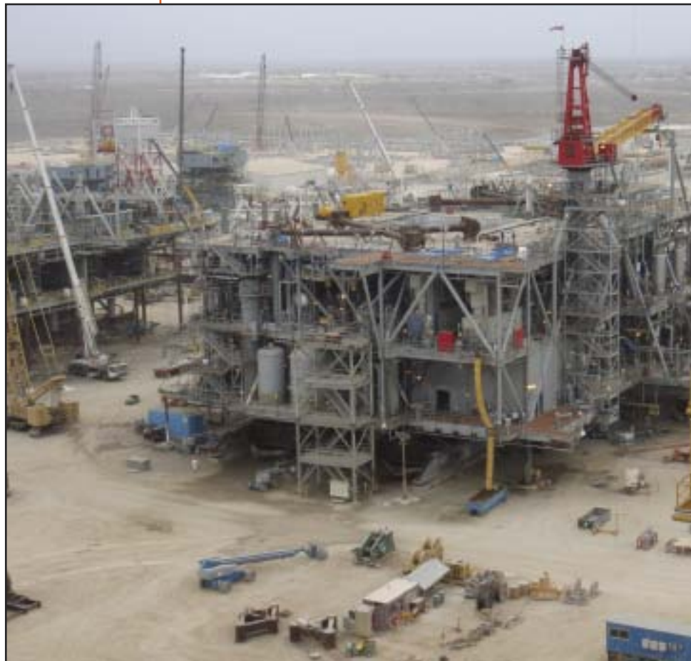
Figure 1: Perdido topsides are constructed at Kiewit Offshore Services in Ingleside, Texas. USCG photos by CWO Earl Schlemmer.
