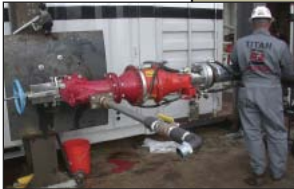
Installation of the viscous oil pumping system. Photograph courtesy of Titan Maritime.
