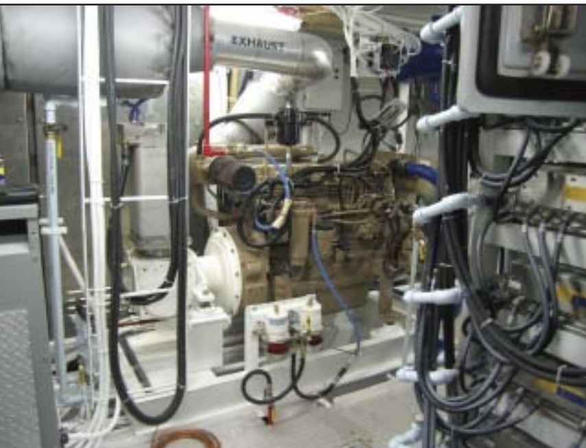
The engine room on a hybrid drive vessel showing the propulsion generator. The cabinet on the right holds propulsion control electronics.
