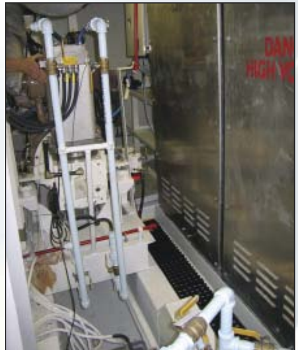
The stainless steel cases on the right-hand side house large battery banks on this hybrid vessel. All photos courtesy of RiverQuest, Pittsburgh, Pa.
