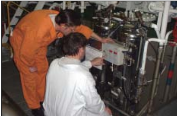
An environmental compliance plan must incorporate detailed procedures to ensure the proper maintenance, repair, and operation of a ship's oily water separator, as well as adequate monitoring and underway testing to ensure that the company's compliance policies are being followed. Photograph courtesy of Marlins™ 2007.
