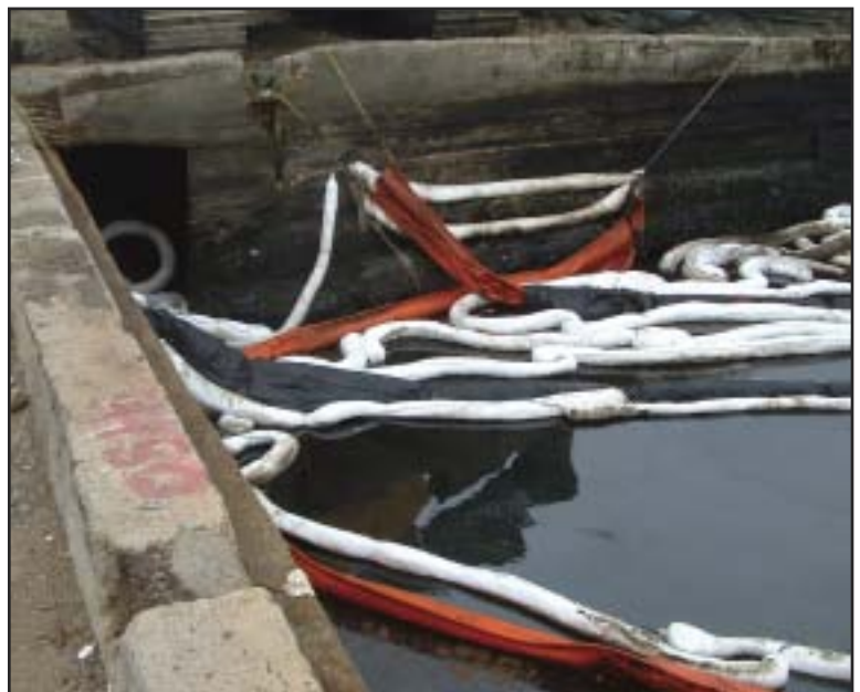
On-site example of excessive use of soft boom during a waterfront remediation project. Once discovered, the USCG assisted contractors toward creating a static hard boom containment procedure that required a minimal amount of soft boom to direct recovery operations. USCG photo by MST1 Joshua Doud.
