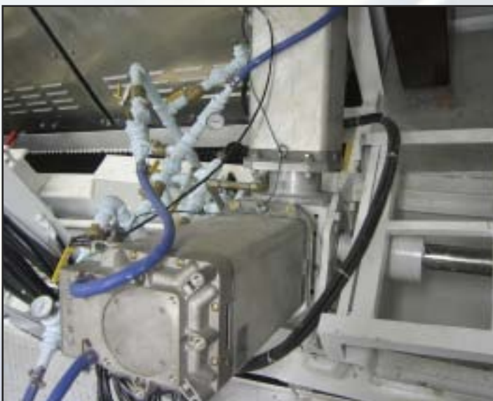
Twin Siemens propulsion motors joined together in a combining gearbox. The propeller shaft emerges to the right.
