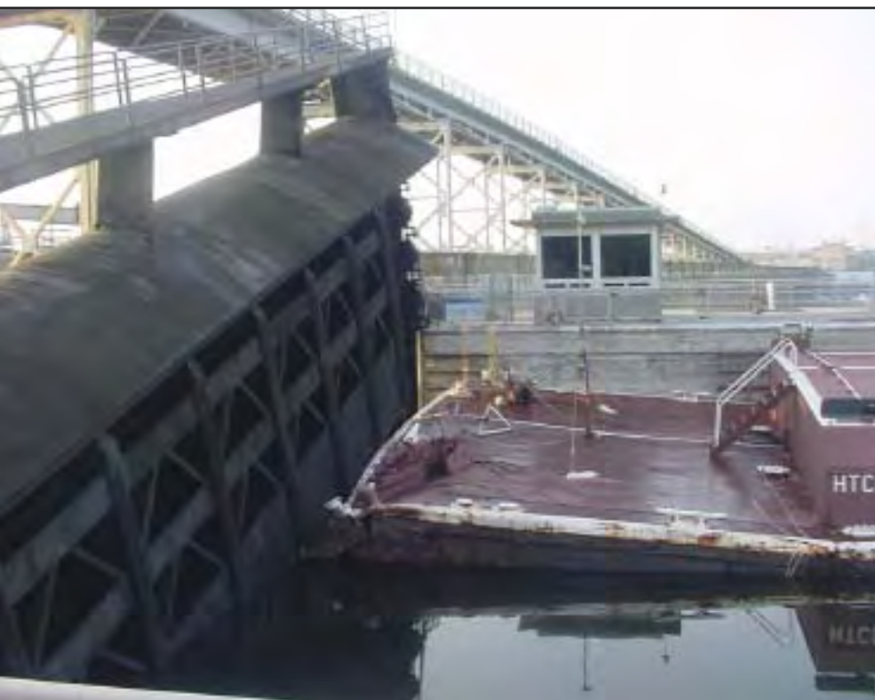
Figure 1: Barge HTCO-3016 pinned beneath the Wilson Lock/Dam upper main lock gate. USCG photo by CWO3 Tim Smith.
