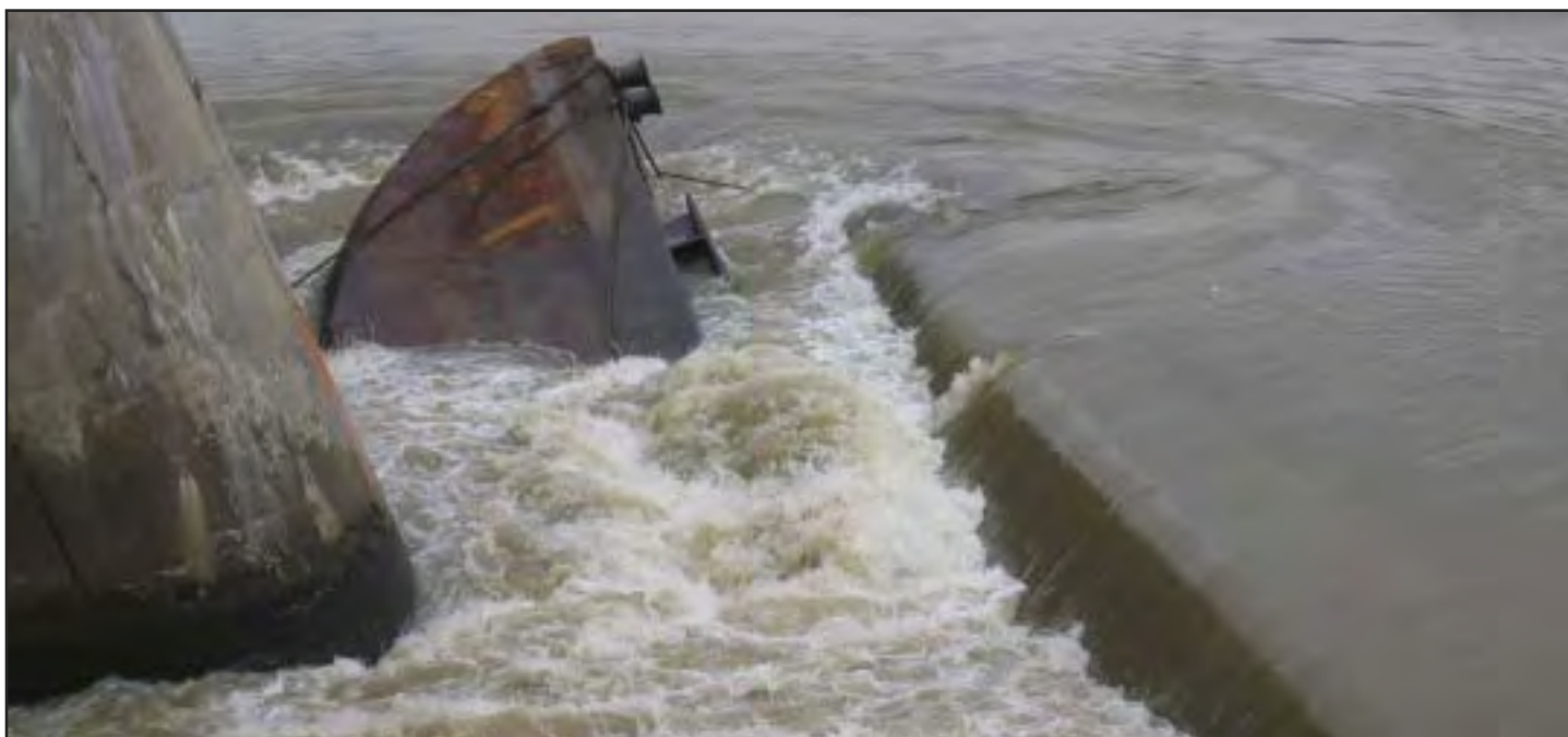
A sunken barge broken from the tow, jammed against the Montgomery Dam pier. USCG photo by LTJG Jesse Garrant.
