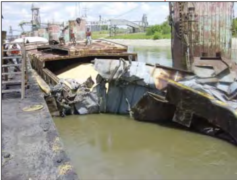
What's left of a hopper barge after an allision with the Eads Bridge on July 6, 2005. The vessel was traveling southbound on the upper Mississippi River at mile 179 as part of a 15-barge tow when it hit a bridge and broke away from the tow. USCG photos.
