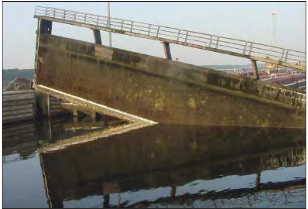
Figure 2: Wilson Lock/Dam upper main lock gate lifted from its track. USCG photo by CW03 Tim Smith.
