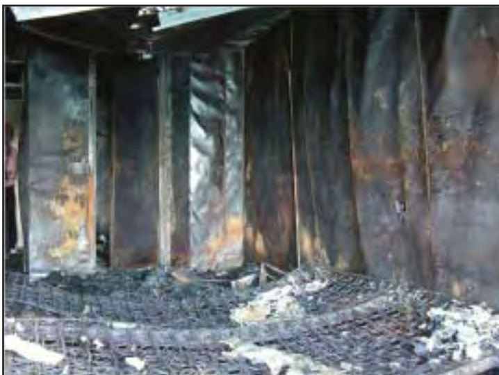
Figures 4a and 4b: The mist system was working properly in the stateroom above. The stateroom below is the only one where the mist system didn't work. USCG photos.
