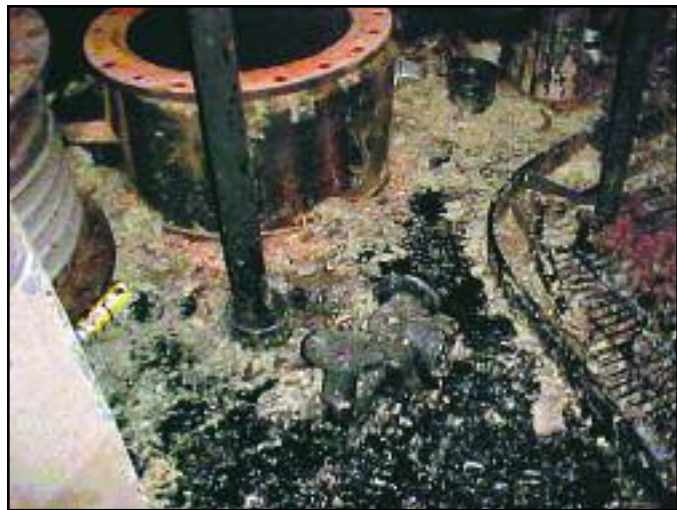
Residual oil on deck in the vicinity of the incinerator exhaust stack of the 03 level of the engine room. Fire damage is visible in the surrounding area. USCG Photo.
