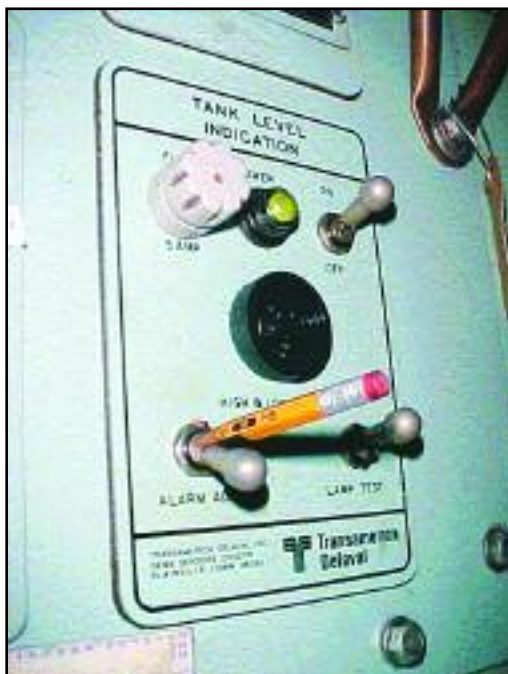
A pencil wedged into the High Tank Level Indicator audible alarm panel. Position of pencil holds switch in "Acknowledge" position. The alarm would never sound to warn of a high tank level when the switch was in this position. USCG Photo.
