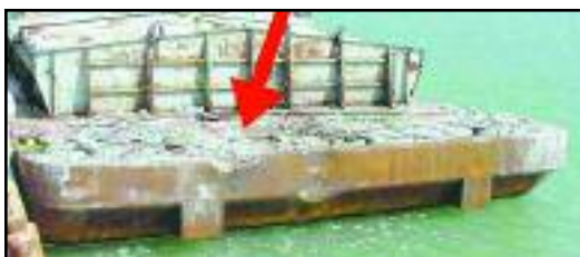
There was some damage to the alliding barge, but no flooding. USCG Photo.
