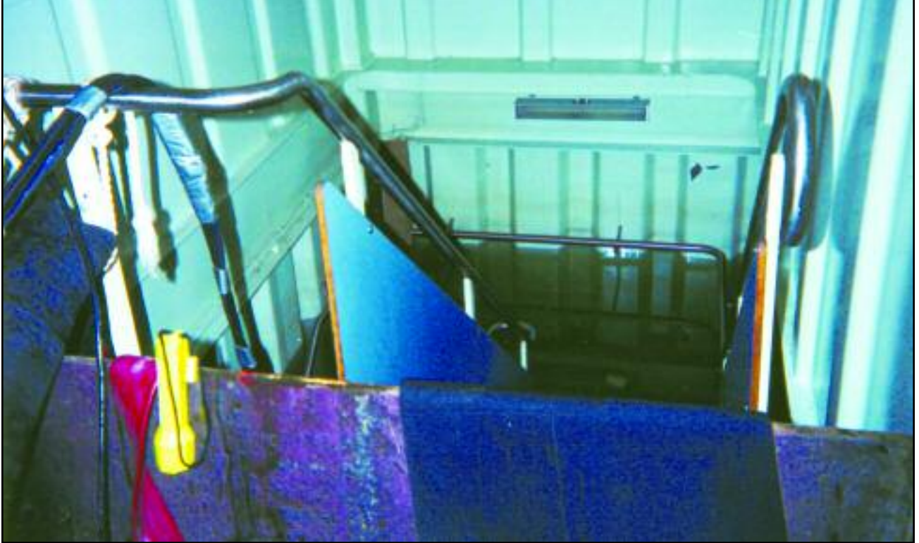
Figure 1: A shot of an interior stairway, showing water level. USCG photo.
