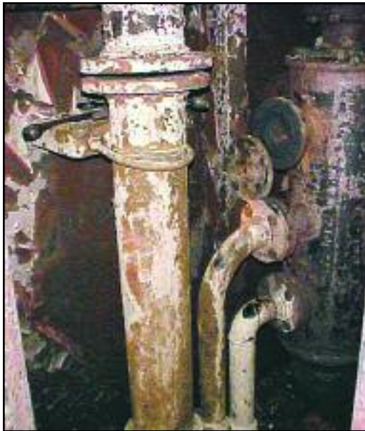
Five-inch drain line from the HFO fuel tank vent collection chamber on the 03 level of the engine room. USCG Photo.
