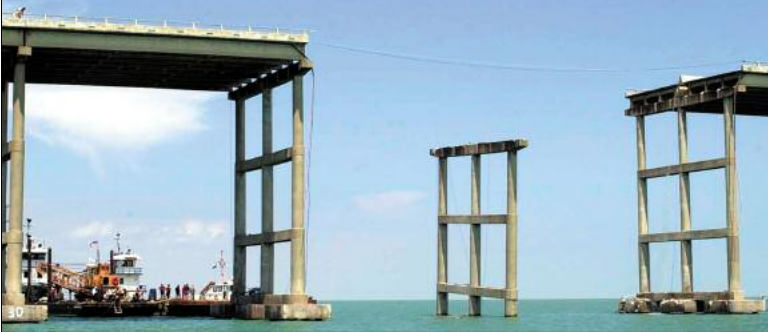
Coast Guard Cutter Mallett crewmembers and Department of Public Safety personnel survey the damage done to the Isabella Causeway near South Padre Island, Texas, September 15, 2001. A tug pushing four barges allided with the causeway, causing 10 cars to fall into the water. CWO2 Robert Wyman, USCG.
