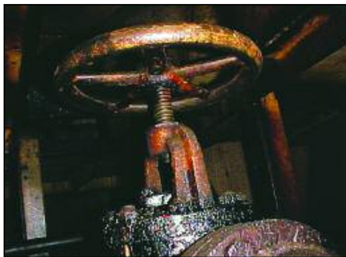
Open discharge valve from HFO (Heavy fuel oil) transfer pump in the lower level of the engine room. Oil and fire damage is visible. USCG Photo.
