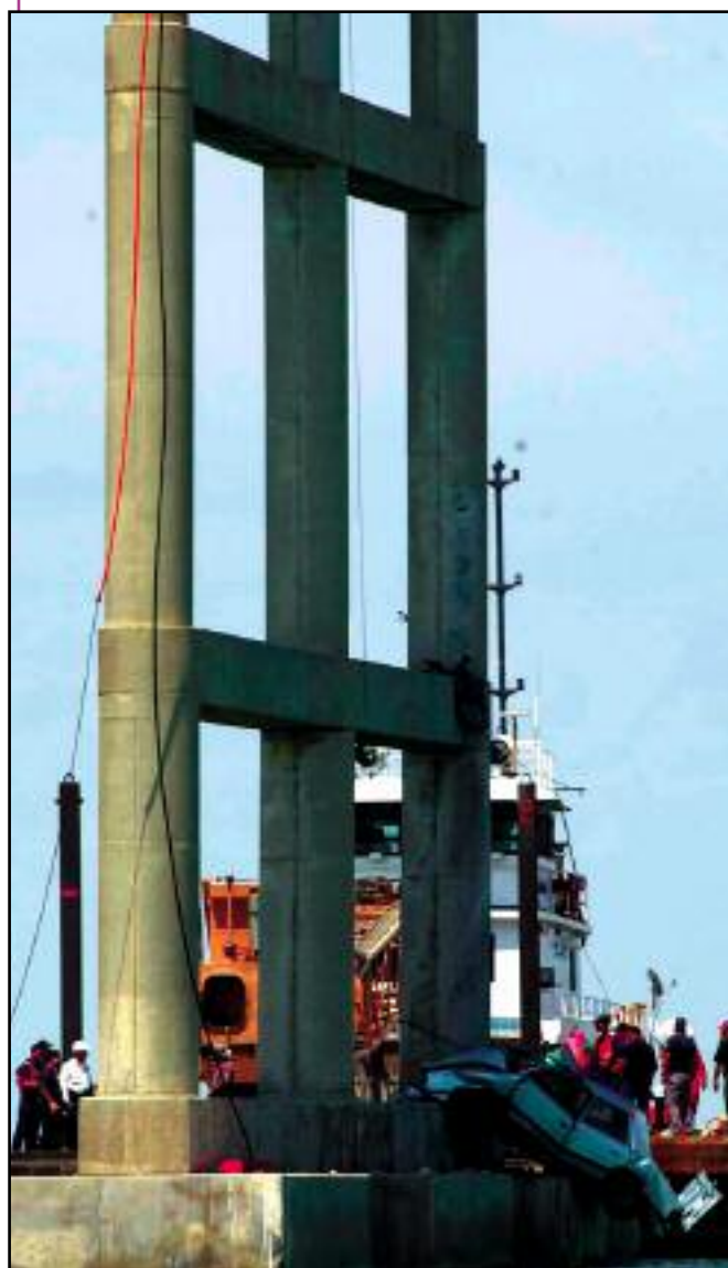
Coast Guard Cutter Mallett crewmembers take a look at a car that was damaged when the Isabella Causeway collapsed September 15, 2001. CWO2 Robert Wyman, USCG.
