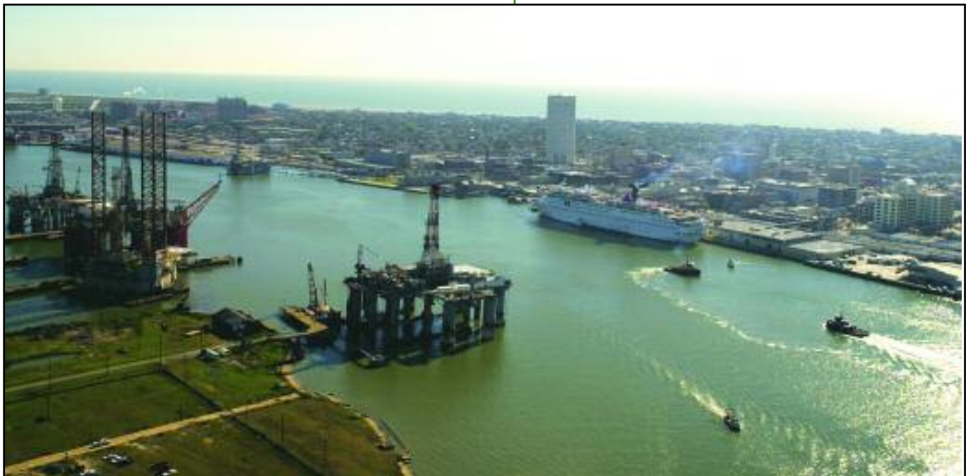
The combined ports of Houston-Galveston see a variety of traffic and service a variety of customers, including tankers, bulk carriers, rigs, cruise ships, barges, and container vessels. Pictured is a segment of the Galveston ship channel during a busy day. PA2 James Dillard, USCG.
