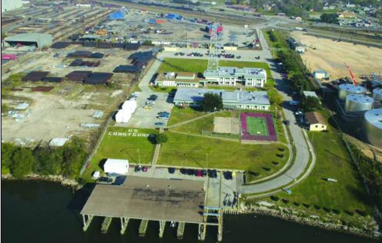
Marine Safety Unit Houston is located on the Houston ship channel. PA2 James Dillard, USCG.
