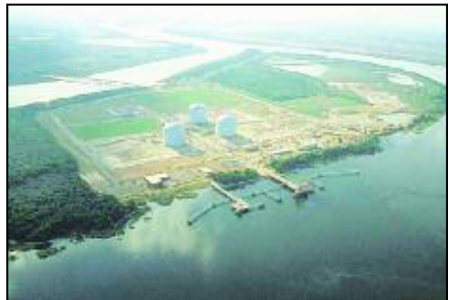
Plans for new LNG infrastructure, marine terminals, and gas carriers are growing, along with the increasing demand for natural gas throughout the world.
