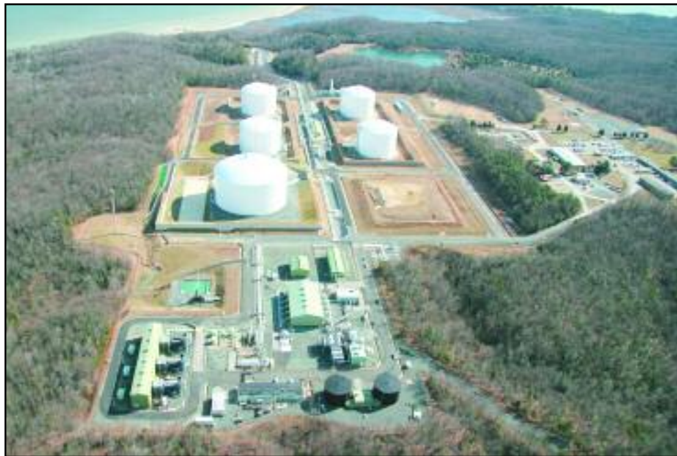
Figure 3: LNG storage tanks, Cove Point facility. Courtesy Dominion, Cove Point.
