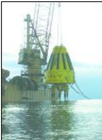
Figure 2: Gulf Gateway submerged turret offloading buoy.
