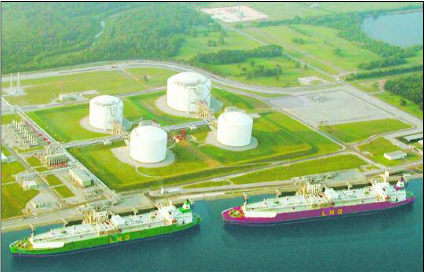
LNG tankers moored at the CMS Trunkline facility in Lake Charles, La.
