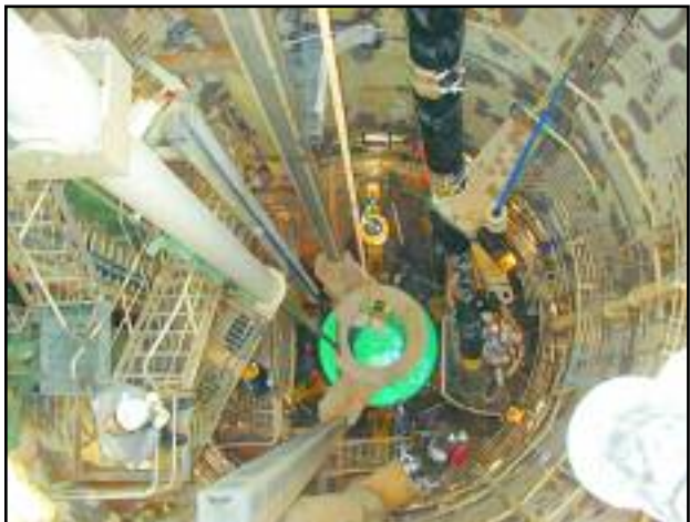
Figure 2: Forerunner deployment during sea/regas trials by builder DSME off the coast of Korea. The STL compartment has not yet received the final coat of paint prior to delivery. Courtesy Captain Mark K. Lane, Excelerate Energy, LLC.
