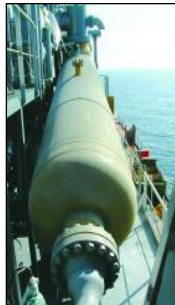
Figure 4: Starboard outboard regasification plant vaporizer as seen from the LNG inlet side. This is one of six vaporizers installed. Courtesy Captain Mark K. Lane, Excelerate Energy, LLC.
