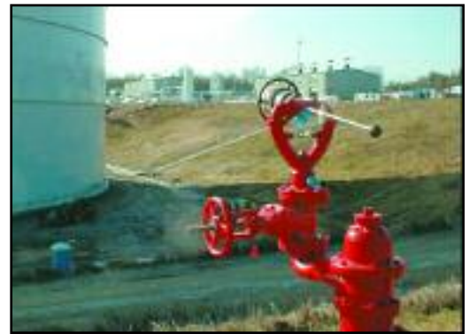
Figure 2. FERC review will assess the coverage of firewater, dry chemical, and deluge systems. Courtesy FERC.
