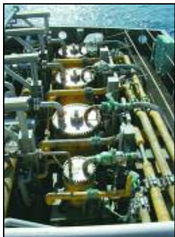
Figure 3: Port side regasification plant high-pressure LNG pumps. Courtesy Captain Mark K. Lane, Excelerate Energy, LLC.
