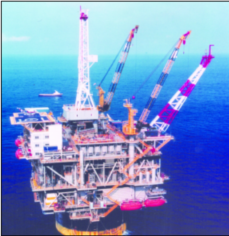
ChevronTexaco's Genesis is the second floating SPAR in the Gulf of Mexico, and the first to accommodate both drilling and production facilities. Genesis' current daily production is approximately 33,500 barrels of oil and 40 million cubic feet of natural gas. Courtesy ChevronTexaco.
