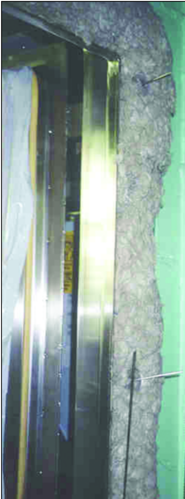
Structural fire protection (SFP) insulation around a walk-in refrigerator, as seen by an MSC engineer during inspection of a vessel.
