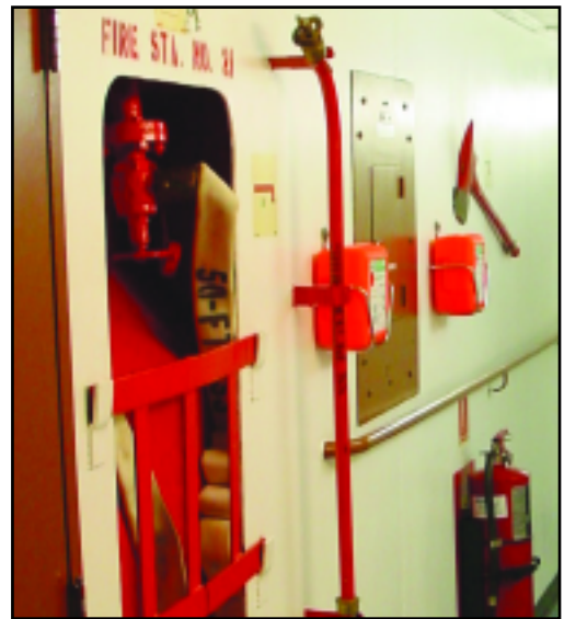
There are many layers of fire suppression systems on commercial vessels: active and passive, fixed and portable, manual and automatic. Every component of this fire station is designed and tested to rigorous standards, and forms a critical part of the vessel's fire safety system. Courtesy U.S. Department of Transportation, Maritime Administration.
