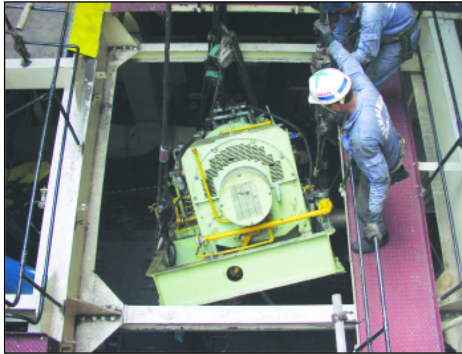
A ship's service turbo-generator is loaded onboard. MSC staff engineers review and approve all aspects of machinery systems, from the type of wire to the location of major machinery, all of which are governed by strict regulatory standards. Courtesy U.S. Department of Transportation, Maritime Administration.
