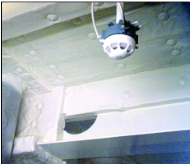
A heat detector on a vessel provides structural fire protection. Courtesy MSC.
