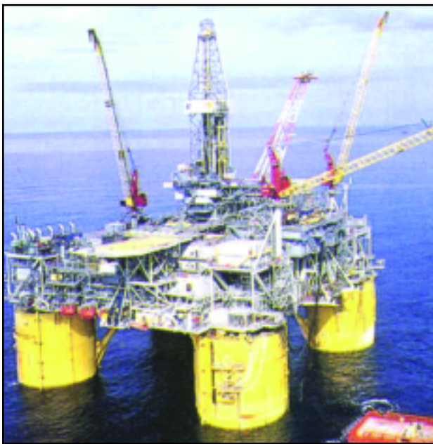
The Ursa, a Shell Oil tension leg platform, located approximately 130 miles southeast of New Orleans. Courtesy Shell.
