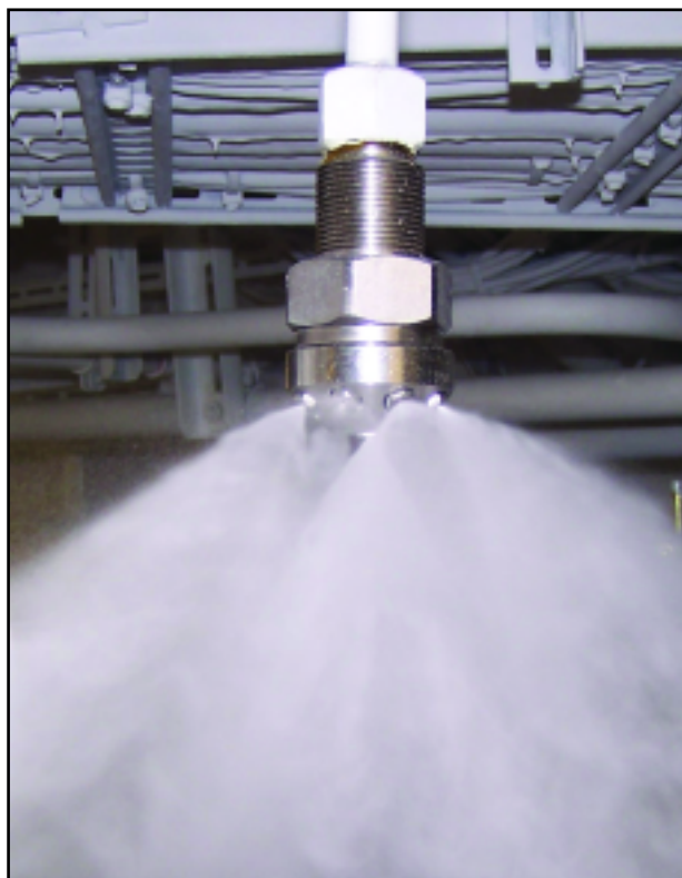
A fixed fire suppression system is another layer in the overall fire safety system. Courtesy MSC.
