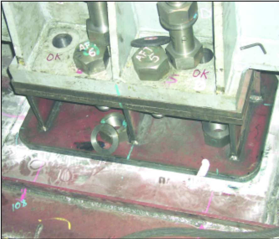
The precise mounting of major machinery is critical to its proper operation and long-term function. This SSTG mounting foot is bolted to a pad that is welded to the deck. MSC staff engineers review and approve all aspects of the design. Courtesy U.S. Department of Transportation, Maritime Administration.
