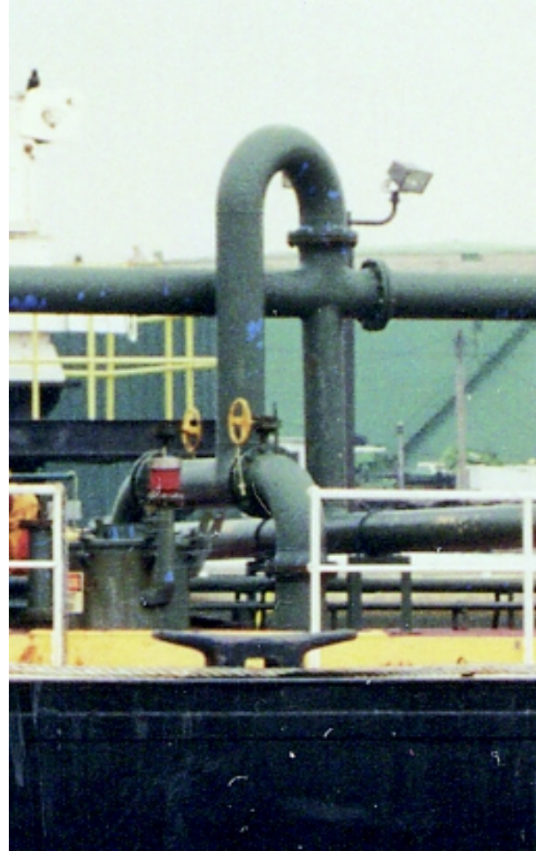
Failure to fully close or open valves provides many examples of reasons for oil spills. USCG photo by Jesi Hannold.
