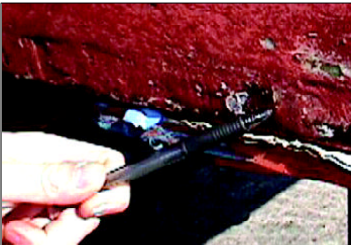
A marine inspector points out the port aft corner of the Elaine B II , which indicates the obvious cross-planked (dead rise) construction of the vessel.
