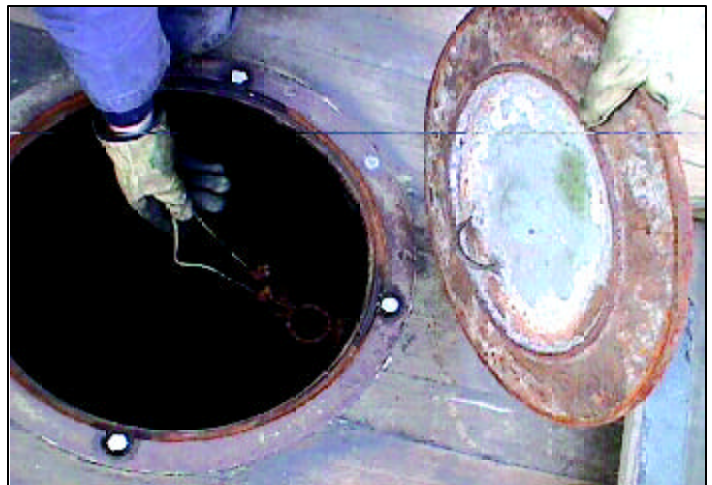
Marine inspectors enter lazarette to examine steering equipment, through hull fittings and planks. Elaine B II 's exterior hatch covers were required to be properly secured to the vessel.
