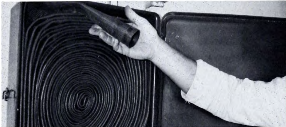
(Above) Hose fittings are held loosely in place by corroded fasteners. (Below) Hoses are missing fittings.
