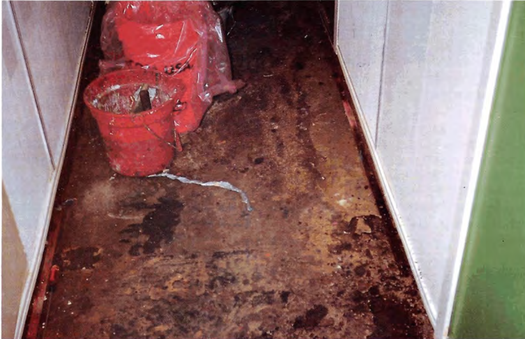
(Below) Deck above #4 fan room after removal of carpet.
