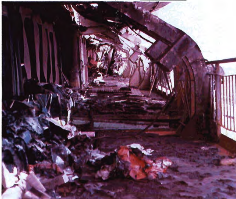
Fire damage on the Angelina Lauro.
