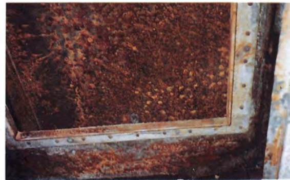
(Below) Galley exhaust duct with access open.
