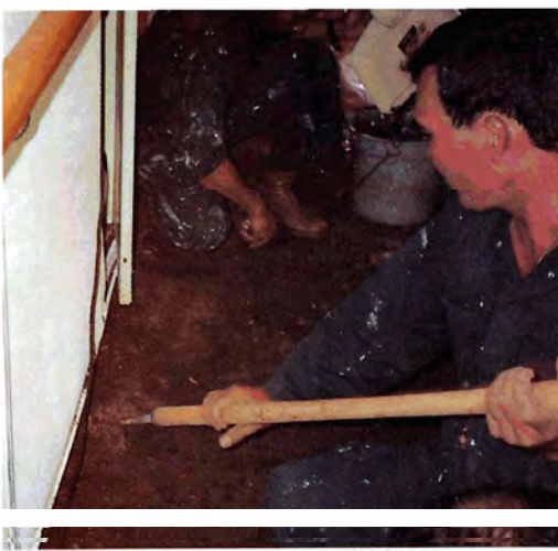
(Left) Insulation is removed from deck above #4 fan room.
