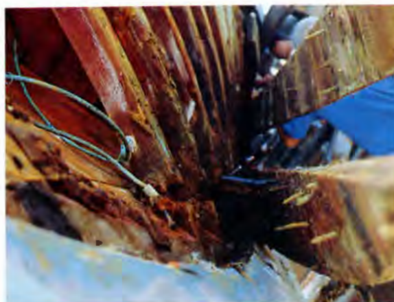
Rotten, broken frame heels were originally fastened to the keel.
