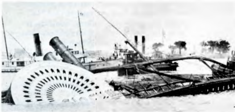
One good reason for regulations -- The excursion steamer General Slocum before and after catching fire and burning in the East River in New York in 1904. More than 950 people lost their lives, including children on a church outing.
