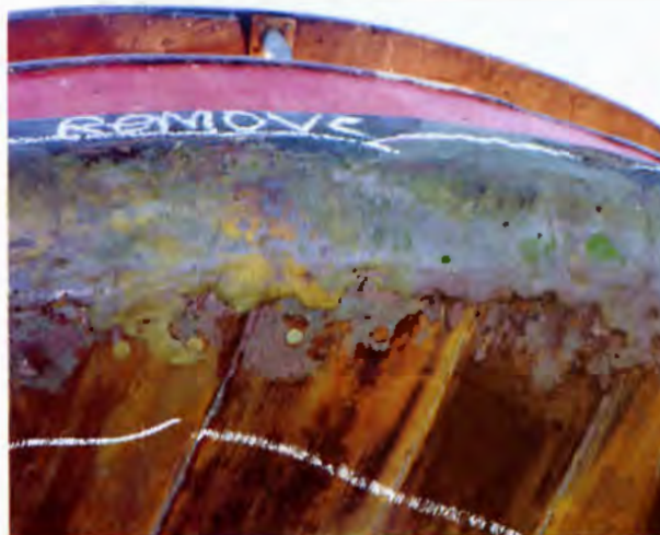
Plank ends filled with water-setting epoxy.
