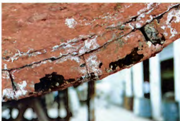
Marine borer damage below waterline at plank ends in way of transom.
