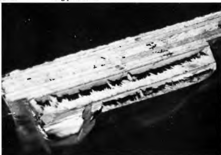
Termites did a job on this timber.
