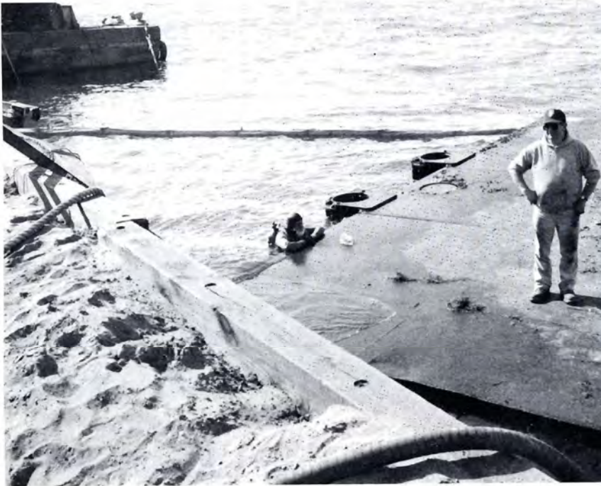
(Left) A diver (center) attached suction and vent hoses to remove fuel from the capsized dredge barge, Rhode Island .
