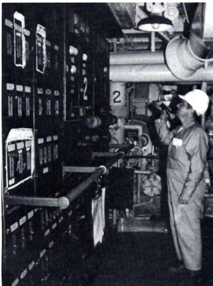
Coast Guard inspector checks electrical generator control board on a commercial vessel. See Proceedings 7-8/92 - p 15.
