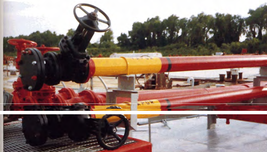
The last one meter of piping is properly color coded: Red-Yellow-Red with "vapor" in two-inch high letters.
