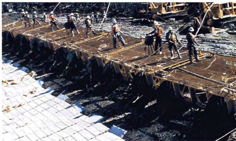
(Above) Concrete mattress is placed along bank of Mississippi River.
